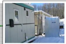
In response to specific client requests, ACPI has developed 3 units suitable for small sewage flows. The **WTS 500, WTS 600 and WTS 1000** units are housed in a custom galvanized metal clad structure – 40" wide, 82" long and 82" high (including C-channel skid).
